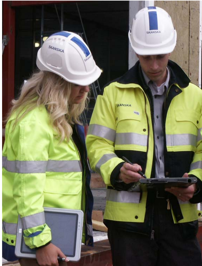
Pic. 1. Tablet computer test at a construction site
